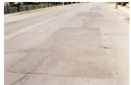
A typical section of repaired pavement
