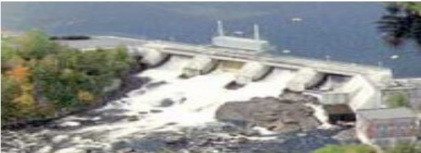
Small Hydro Plant
