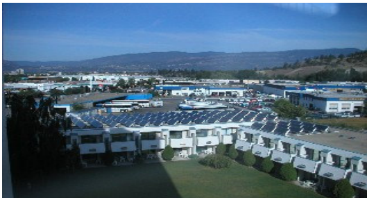
Solar thermal collectors
