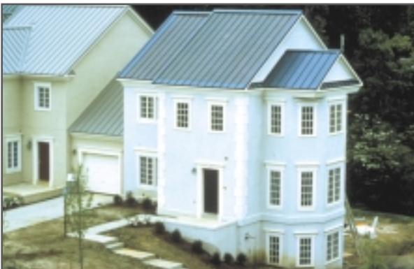
PV rooftop system in Maryland. (© United Solar Systems Corp. USA)
