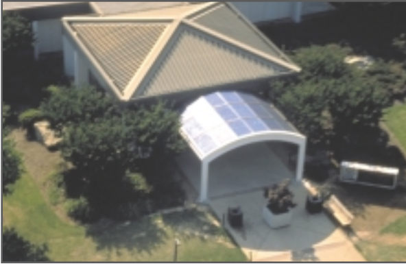
35 kW p PV modules that allow light transmission between the individual solar cells, integrated into the support structure on the entrance of the Olympic Natatorium on Georgia Institute of Technology, U.S.A. (© Solar Design Associates, Inc.)
