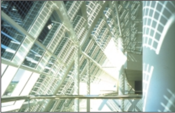
Semi-transparent and dummy modules. The Solar Office at Doxford International Business Park. (© Dennis Gilbert)
