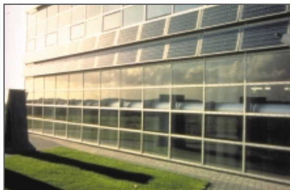
A 4.4 kW p PV power system integrated on the south-east façade and a 9.8 kW p system integrated into the atrium roof of the Brundtland Centre, a low-energy office building in Denmark. (© Esbensen Consulting Engineers A/S)
