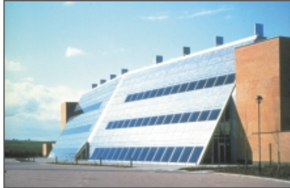
A 73 kW p PV array integrated into a 900 m 2 south facing façade inclined at 60 degrees, of the Solar Office at Doxford International Business Park, in England. The PV system is expected to provide 55,000 kWh of electrical energy per year, representing between one third and one quarter of the expected electrical usage of the building. (© Dennis Gilbert)
