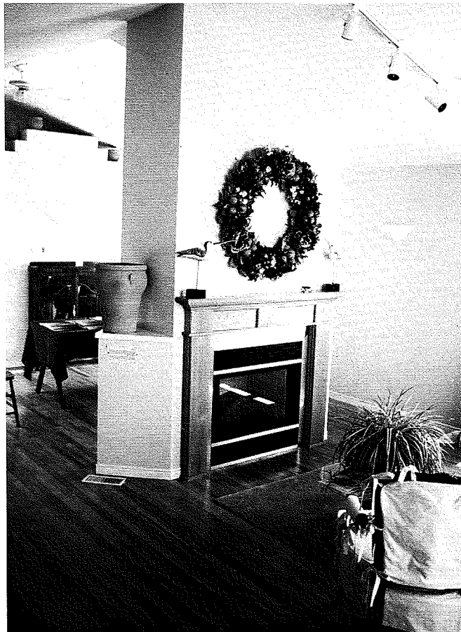
The direct-vent natural gas fireplace in Canada's Green Home features spark ignition and fan-assisted heat delivery. The track lighting visible above demonstrates the overall lighting strategy of the house; spot lights illuminate specific areas rather than the entire room.
