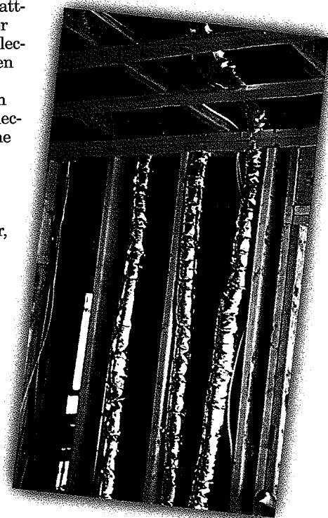
Small insulated air-distribution ducts are flexible and reduce heat losses.
