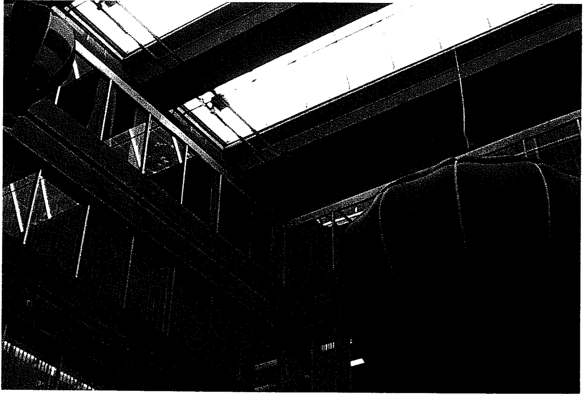
The Southport Office Building in Calgary uses atrium exhaust air to heat the underground parking garage.
