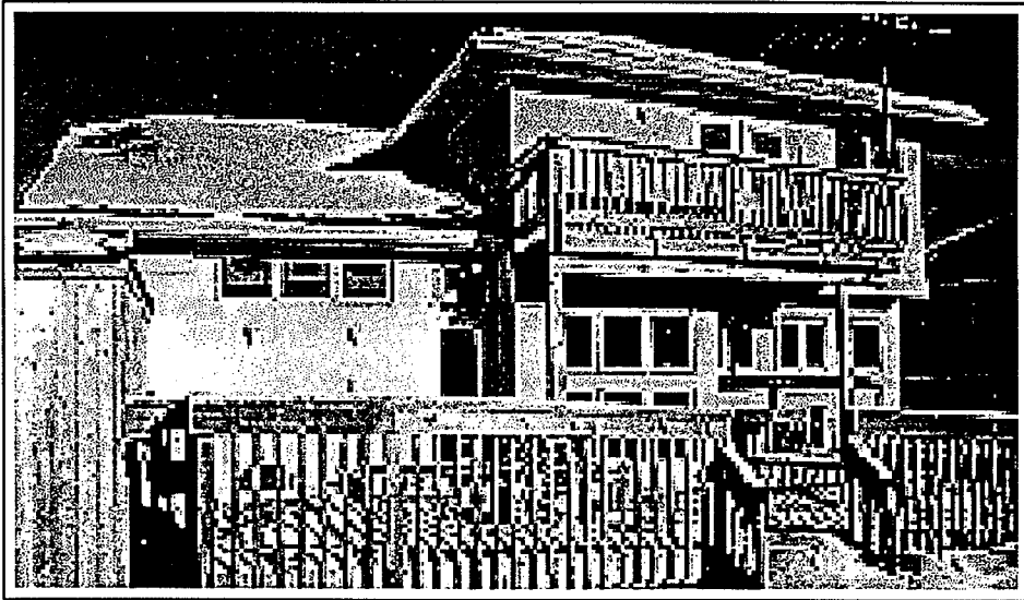
Figure 2.12 Shading of South Windows - Main and Second Floor (B.C. Advanced House) - a change in the dormer roof slope orientation would improve the shading characteristics of the second floor overhangs.
