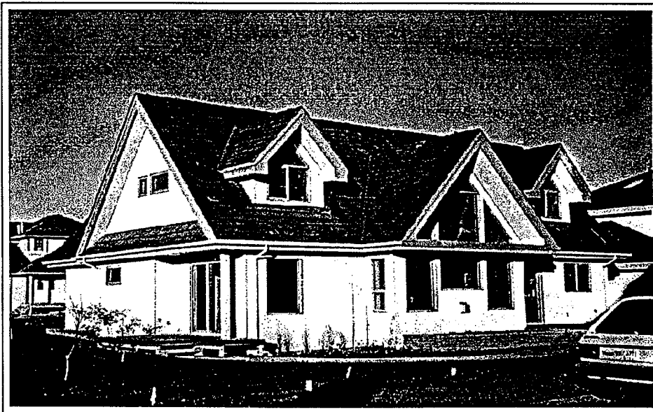
Figure 2.12 Shading of South Windows - Main and Second Floor (B.C. Advanced House) - a change in the dormer roof slope orientation would improve the shading characteristics of the second floor overhangs.
