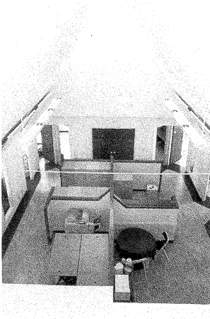
Figure 5.10: Photograph of Second Floor Interior Office
