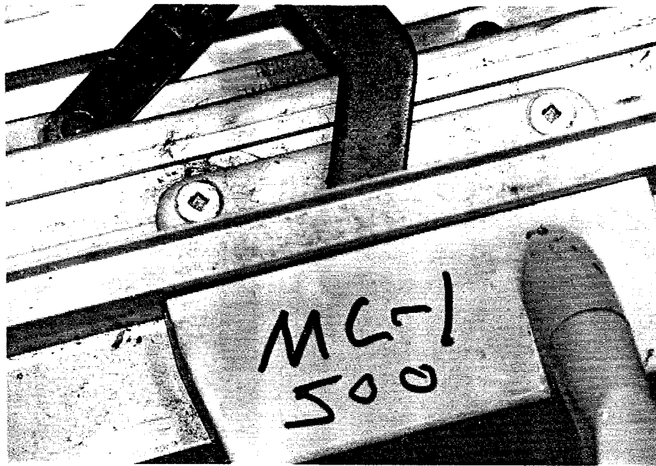
PHOTOGRAPH NO. 3: MC-1 (Aluminum-casement) after 500 cycles - Sill (exterior view) - Weatherstripping wear
