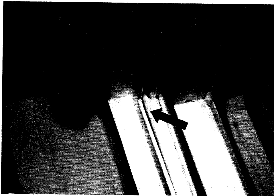
Photograph 2: Sash warping, lower left corner (specimen 8)
