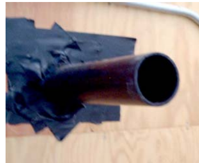
Figure 9 – Exhaust Vent Termination Sample No. 04-06-M278-5
