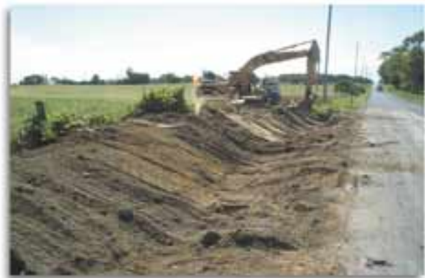
CMP excavations in Port Hope.
