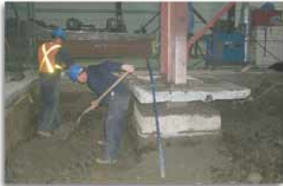
Excavation around a building column at the Anvil Way site.
