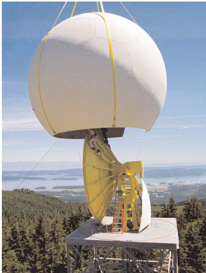
The construction of this Doppler radar on Mt. Sicker, B.C. means Canadians in Victoria and its environs benefit from longer warning times when severe weather is headed their way.
