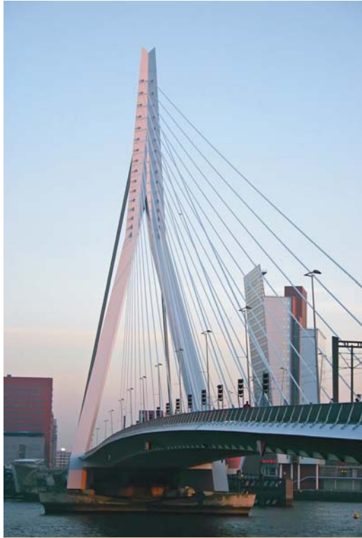
The Erasmus Bridge in Rotterdam.
