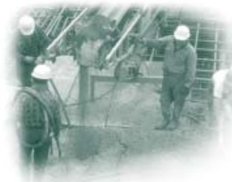
The use of EcoSmart™ concrete in construction projects has the potential to reduce carbon dioxide emissions by substituting fly ash and other materials for the cement generally used in concrete.
