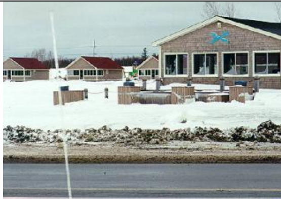
Photo 10. Wetting line at Shediac Bridge.
