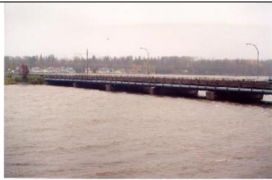
Photo 29. Bouctouche bridge, October 29, 2000.
