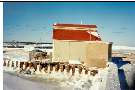
Photo 16. Wetting line on tide-gauge building.
