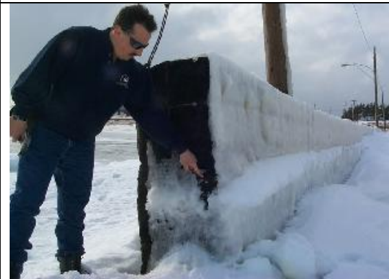
Photo 18. Marking the water level at Cap-Pelé.
