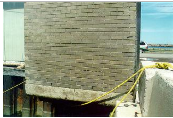
Photo 17. Record water levels at Pointe-du-Chêne.
