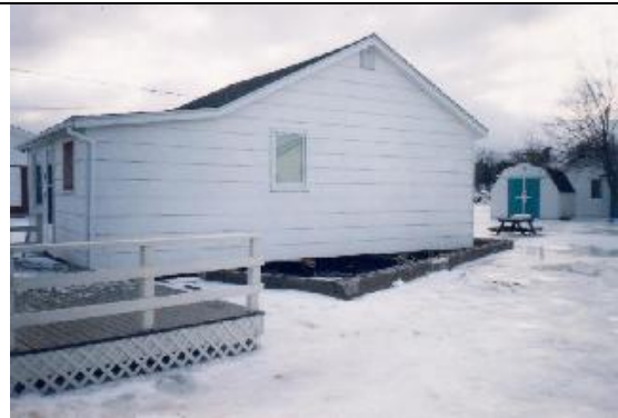
Photo 15. House off foundation in Pointe-du-Chêne.
