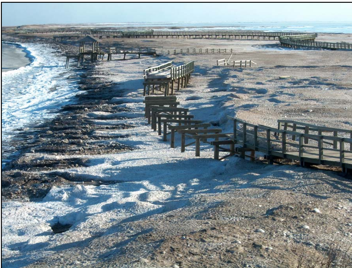
Figure 11. Damaged boardwalk and frozen slush at La Dune de Bouctouche, following storm of December 27, 2004 (Photo: R. Daigle).
