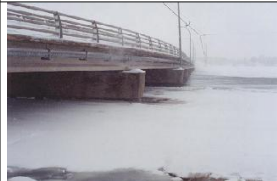
Photo 28. Bouctouche bridge, February 6, 2001.
