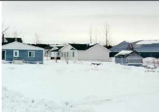
Photo 11. Wetting line at Shediac Bridge.
