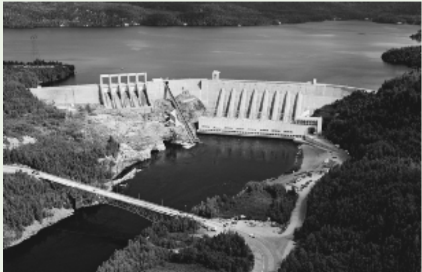
A changing climate may affect the level of hydroelectric reservoirs, leading to financial implications.
