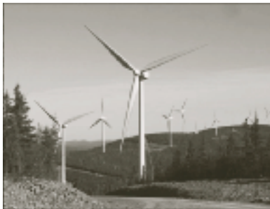
A wind farm on Mont Miller in Quebec.
