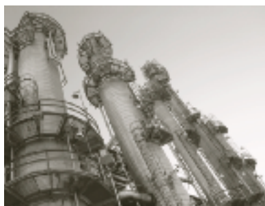
An ethanol production plant in Ontario.
