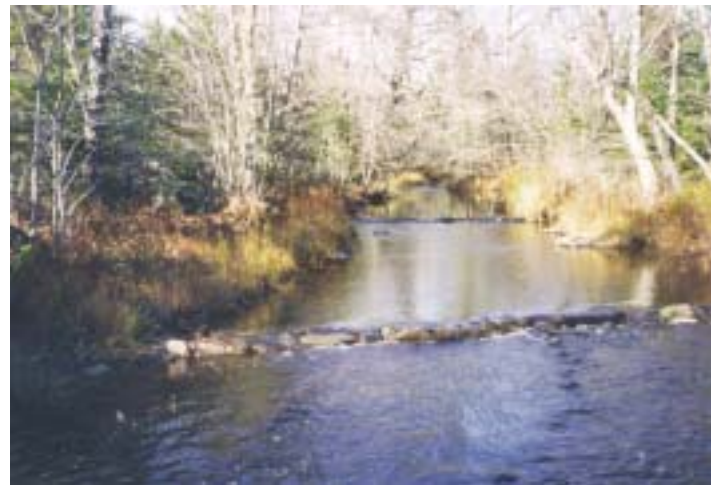
Habitat enhancement: rock sill structure.
