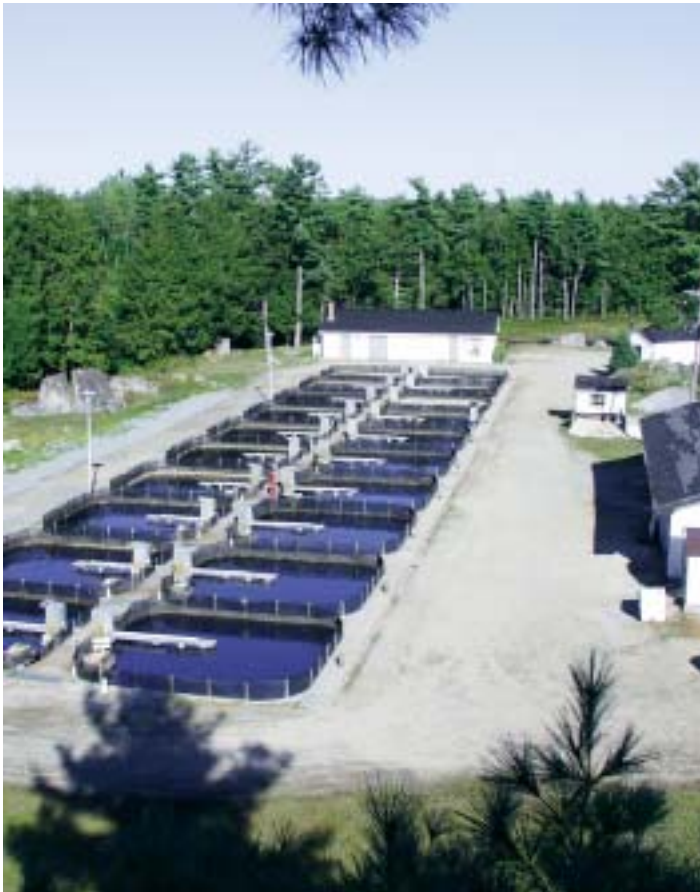
Mersey Biodiversity Facility upper ponds and culture and research buildings.
