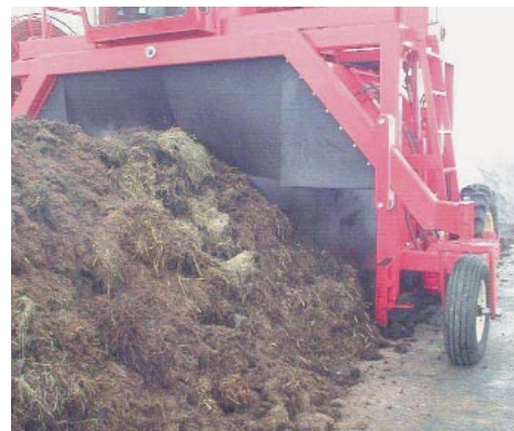
Waste to be composted with a windrow turner (before composting/beginning of process) Westmorland Institution's composting facility
