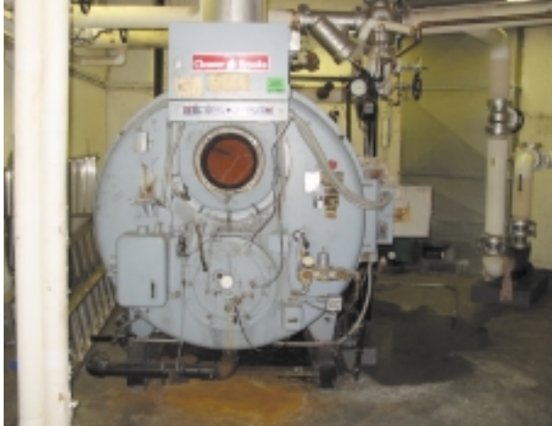
Old furnace system at Hendry House
