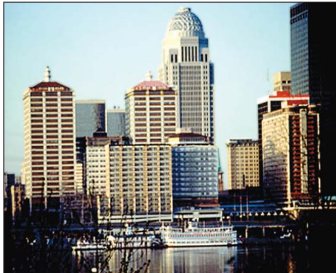
Figure 5: World's Largest GSHP Systems installed in a Building Cluster at the Galt House East Hotel and Waterfront Office Buildings in Louisville (KY), USA.
