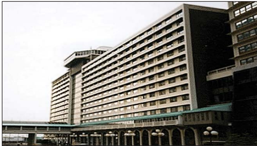
Figure 15: GSHP System in a Commercial Buildings.
