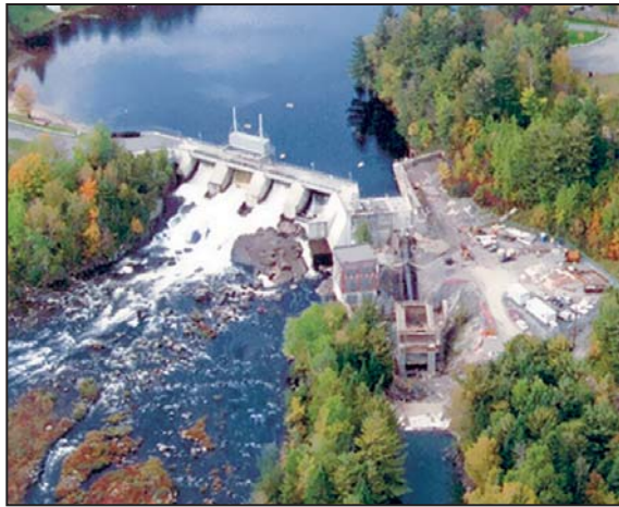
Figure 6: Small Hydro System.
