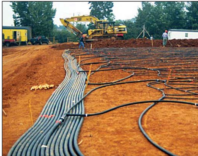
Figure 12: Ground-Source Heat Pump System.
