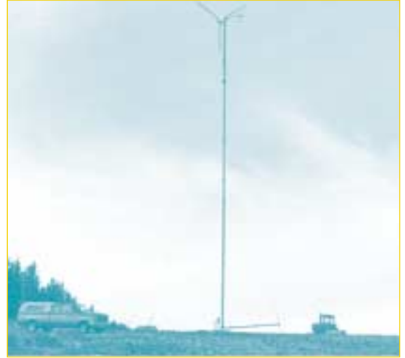
▲ A small stand-alone wind energy system can supply power to both the farm and residence. (Information and photo courtesy of Nor'wester Energy Systems Ltd.)
