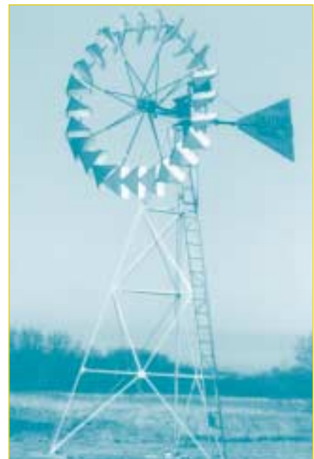
▲ Mechanical water pumping system.
