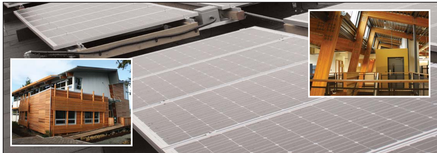
Main: The solar panels on the roof of the Operations Centre supply 20 per cent of its energy needs. Left and Above: Exterior and interior views of the Operations Centre.
