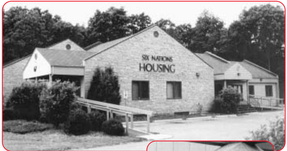
Above is an example of a Native Stone facade.
