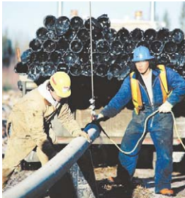
Dene Thla First Nation member participates on pipeline construction
