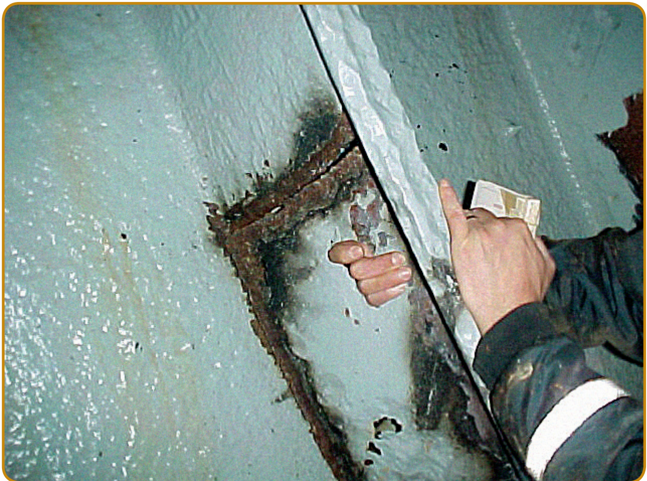
Corroded frame
