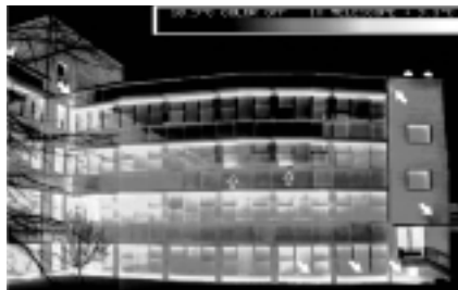
PWGSC uses the latest infrared technologies to detect problems in building envelopes.
