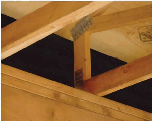
Wood framing for building houses (Natural Resources Canada Library).
