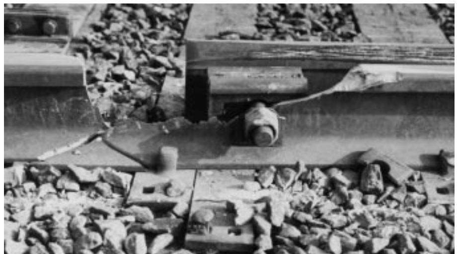
The broken rail at the point of divergence
