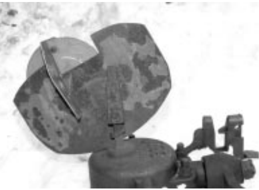
Switch target and tip assembly from 36-D switch at the main-track crossover at Mile 65.1 immediately after the accident, as viewed in the direction of travel by the VIA train crew
