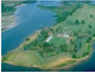
Fort Lennox, Quebec Early 19th Century Fortifications
