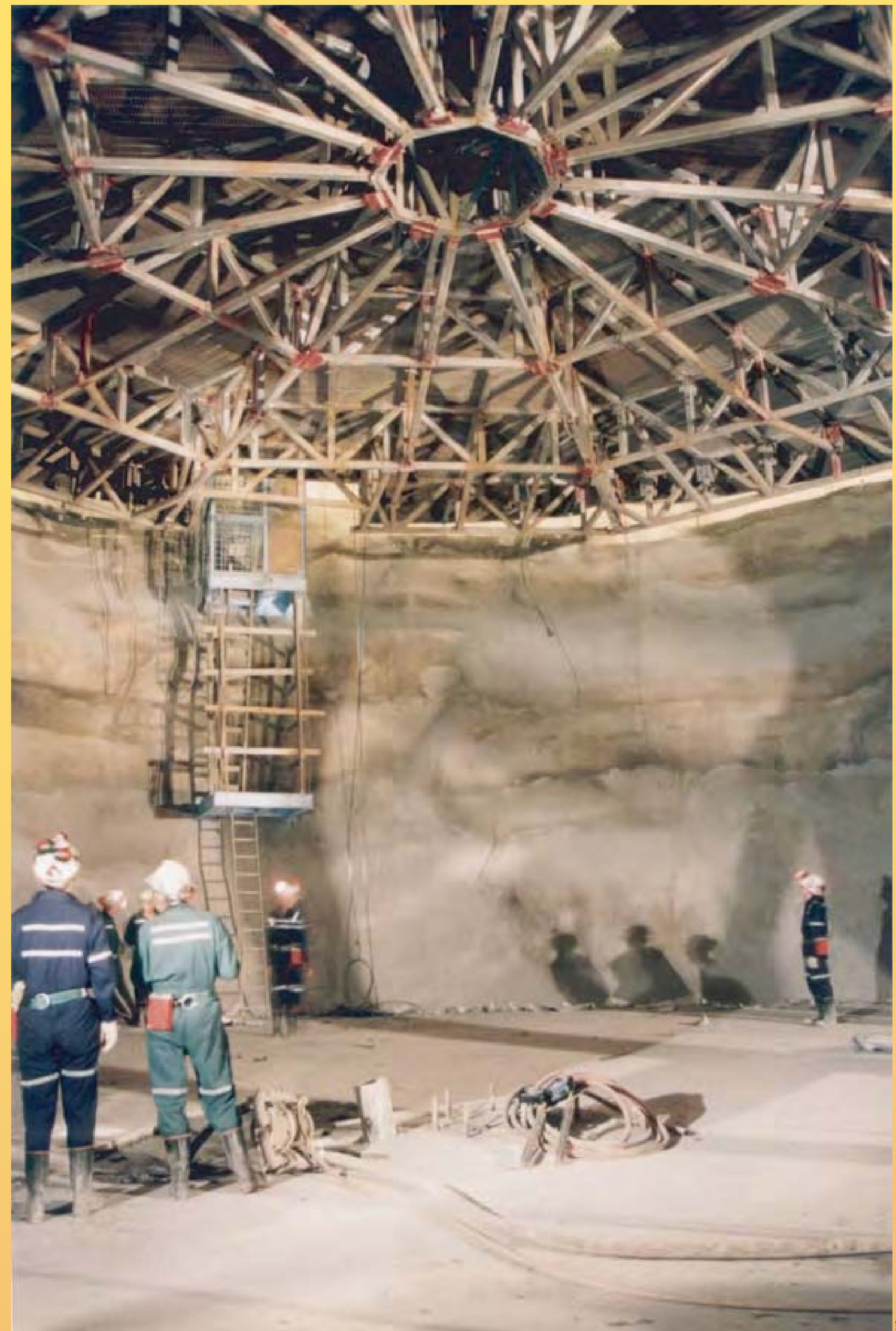
The excavated cavity, two kilometres (1.2 miles) below Earth's surface, required the latest in mining techniques.
