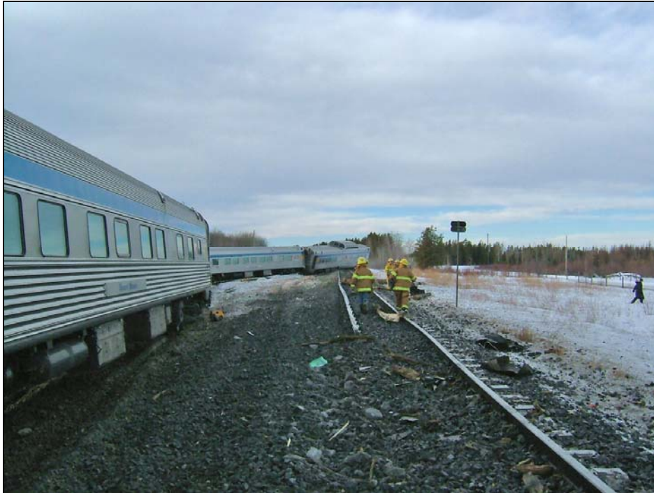
Photo 2. View of the derailment and associated track damage looking eastward from the crossing
