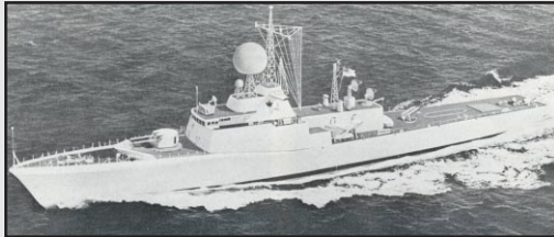
The St. Laurent design was the basis for a general-purpose frigate (above) that was designed in the late 1950s. Twenty metres longer and 1,000 tons more in displacement than the 205-class, the GP ship was intended to become the fleet's air warfare frigate. The GP frigate program was ultimately scrapped, but its design in turn influenced the design of the DDH-280 Iroquois class commissioned into service in the 1970s and modernized (top) in the 1990s.
