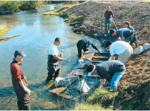
Upper Thames River Conservation Authority
