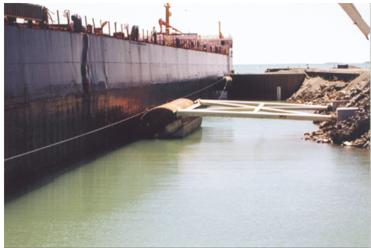
Photograph 1. Starboard side of damaged vessel showing longitudinal deflection of hull
