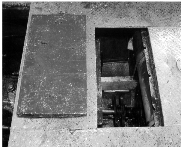
Photo 3 Hatch opening in main deck with no sealing gasket or means of securing flush wooden cover.
