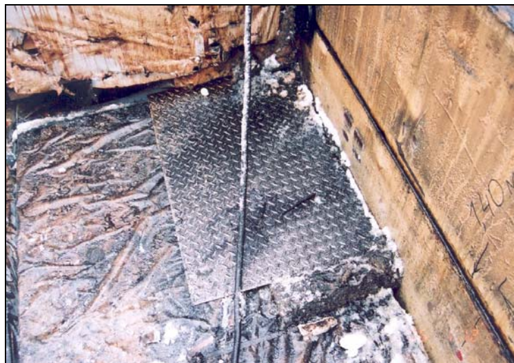
Photo 2. Hatch coaming and aluminum plate on top of a wood bundle adjacent to the welding area
