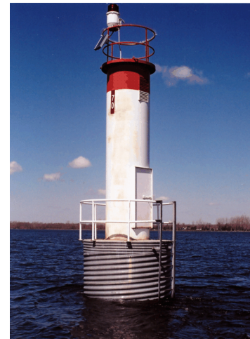
Photo 3. Typical crib light
