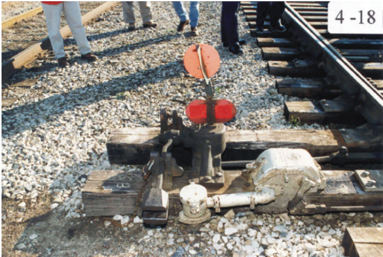
Figure 3 - West crossover switch, Mile 46.72, lined and locked in the reversed position
