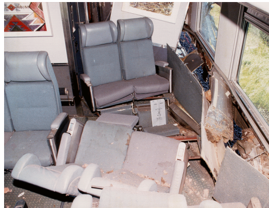
Figure 4—Inside damage from same impact
