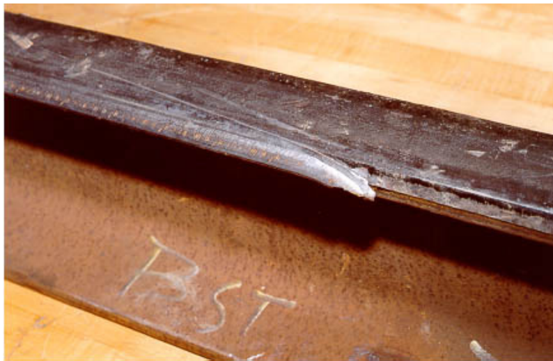
Figure 2. Witness marks and sheared flow lip on the gauge side of the north railhead
