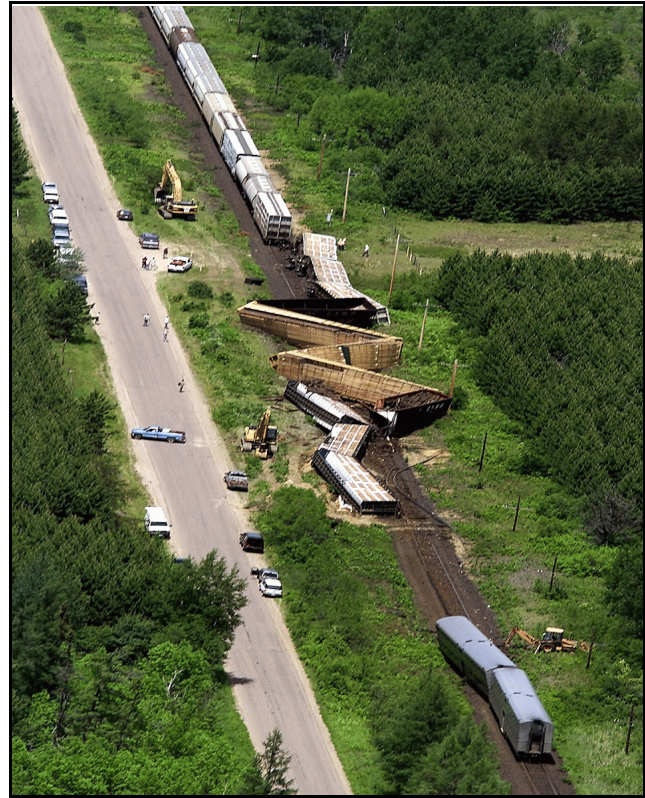
Figure 1. Aerial site photograph facing westward.
