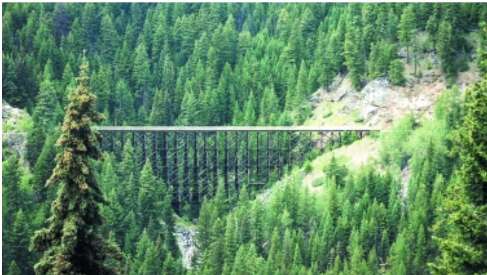
The Chrysler Trestle, Kettle Valley Trail.
