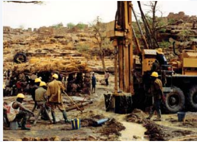
photo: TECSULT (Groundwater Drilling-Mali)
