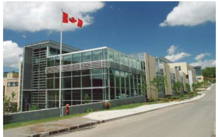
Aerospace Manufacturing Technology Centre
