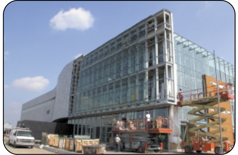
Construction of the NRC Aluminium Technology Centre is near completion.
