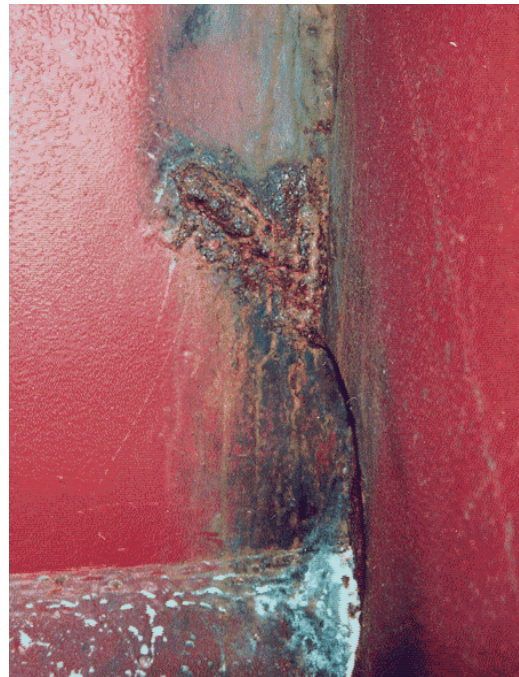
Photo 6. Membrane 171½, tribord
