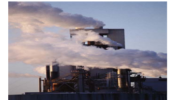
Utilities / Services publics $159.1 M
