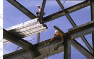
Construction / Construction $477.5 M
